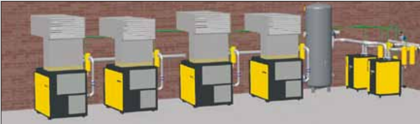
Compressed air supply system with separate components
